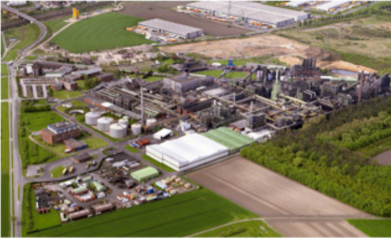
Evonik Degussa Chose HIMax for its Ability to Maintain Non-Stop Operation During Maintenance Work or Software or Hardware Changes.
